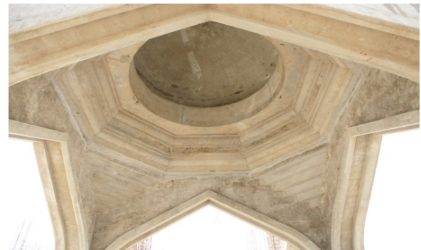
(b) Typical detail of 99 domes of Allahabad Mosque in Fair Face Concrete
