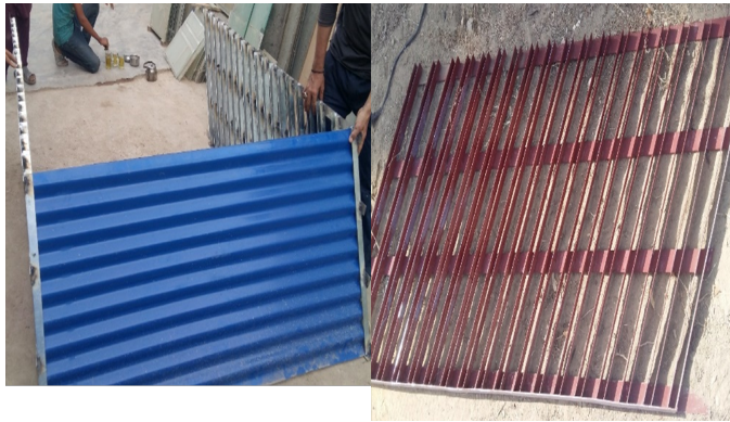
Fig. 2: Construction of the frame for holding plate
