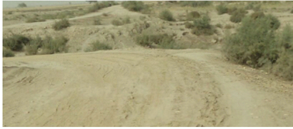
Fig. 1: Failure of a local road embankment during flood in 2010
