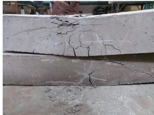
Fig. 10: Cracking in 50% RCA beam
