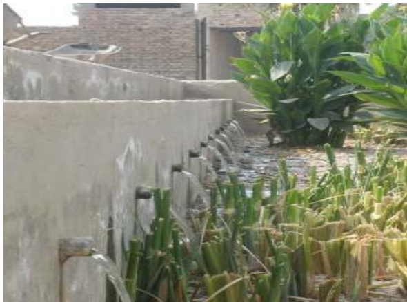
Figure 2: Water flow arrangements of CW Majeed Kerio
