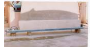
Fig. 8: A bulkhead system fabricated for pre compression
